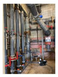
The **Administration Building** HVAC system is antiquated, inefficient, beyond its useful life, and should be replaced. The estimated cost for replacement is \$270,000. Also the aging electrical equipment in the mechanical/electrical room should be considered for replacement. The
