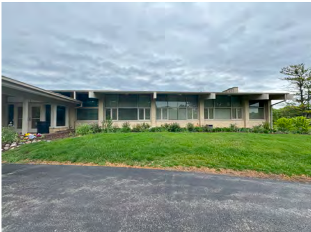
Exterior Exhibits Significant Wear
