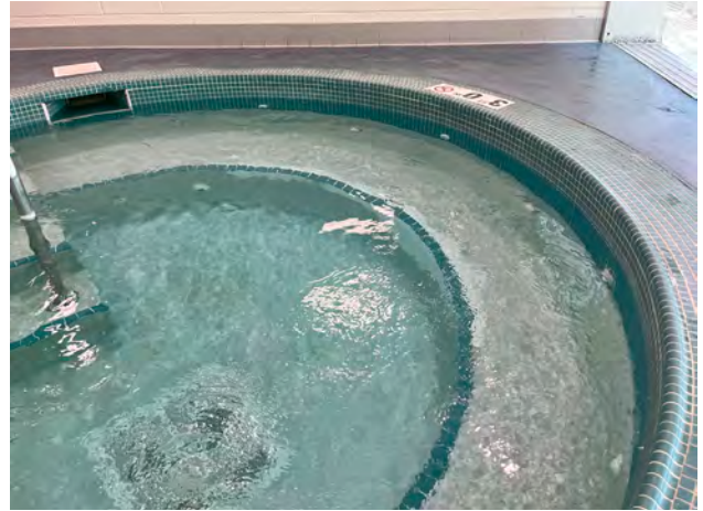
Splash Central - Peeling Spa Finish
