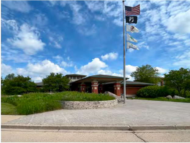
Exterior - Limited Signage
