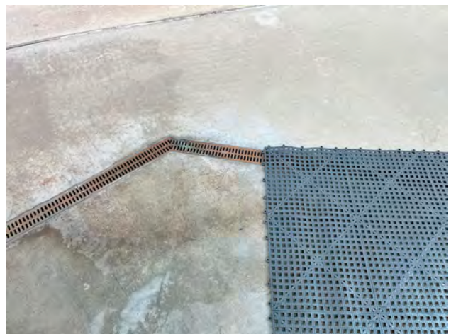
Splash Central - Pool Deck Mats Covering Trench Drains
